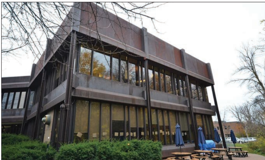
The east side of the building features varying widths of mullions and Cor-Ten cladding, reminiscent of the John Deere building.
