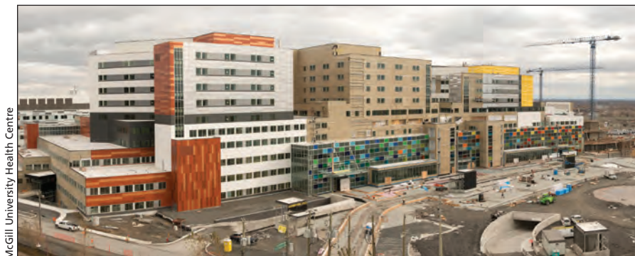
The new 223 000 m 2 superhospital in Montréal will be the largest in Canada. It includes 500 single-patient rooms and two emergency departments.
