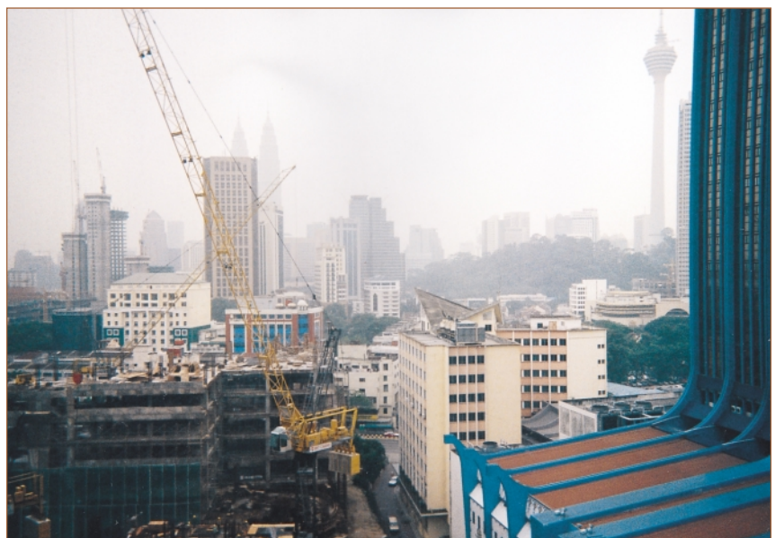
Smoke and haze covered Kuala Lumpur
