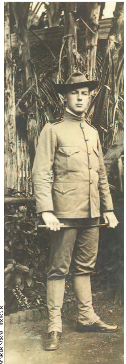
Annadale National Historic Site
