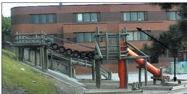
**Fig. 1: An unsafe (above) and a safe (right) playground.** In the unsafe playground, the height a child may fall from equipment is greater than 1.5 m, the surface under the structure is bare earth and the surface on the hillside is concrete, even though it is an area where a child might fall. The equipment at this playground was removed and replaced.
